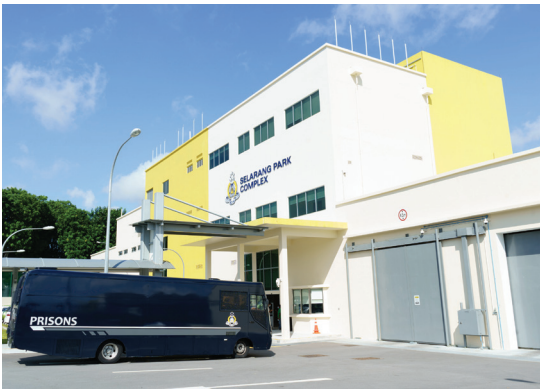
The Selarang Park Complex is an integrated facility that incorporates advanced technology.
