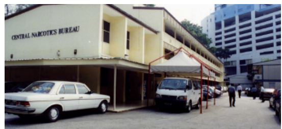
Former CNB Headquarters at Outram Park
